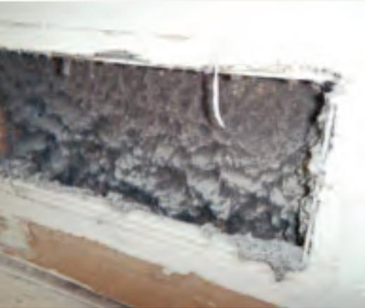
**Clogged Duct:** In extreme cases such as this, ductwork can become totally clogged, totally restricting air flow.
