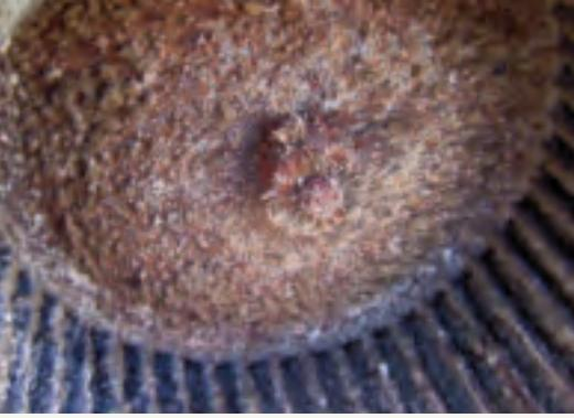
**Dirty Fan:** Blowers such as this can become heavily contaminated and require cleaning for maximum efficiency.
