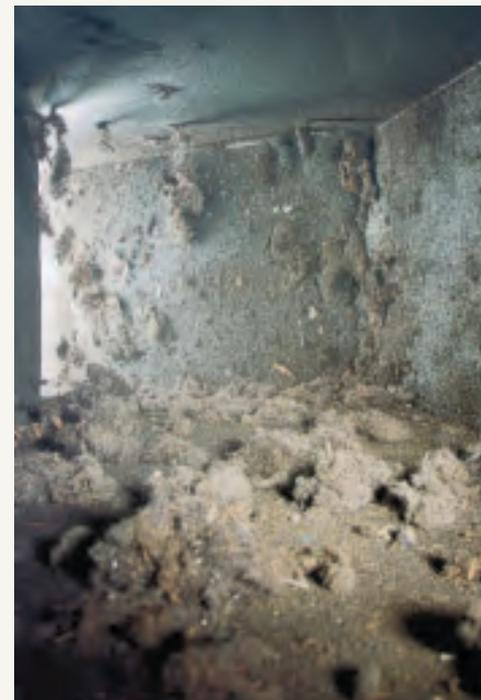
**Dirty Duct:** Accumulations of dust and debris within HVAC ductwork can contribute airborne particulate within a home or commercial building, while also reducing air flow and increasing energy consumption and related costs.
